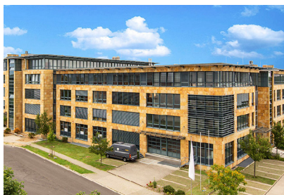
SCAT Europe Headquarters in Mörfelden-Walldorf.
